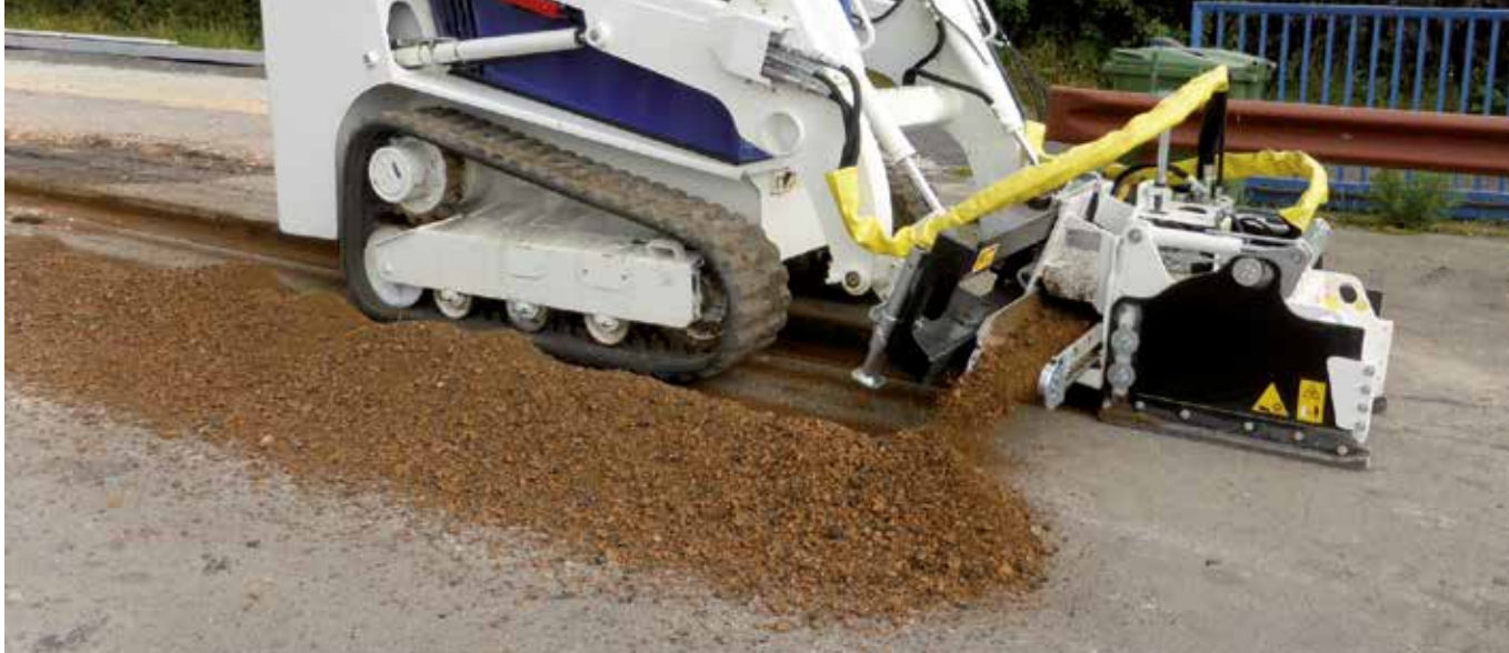
Conveyor belt - the trench is cleared and the material is discharged to the side
