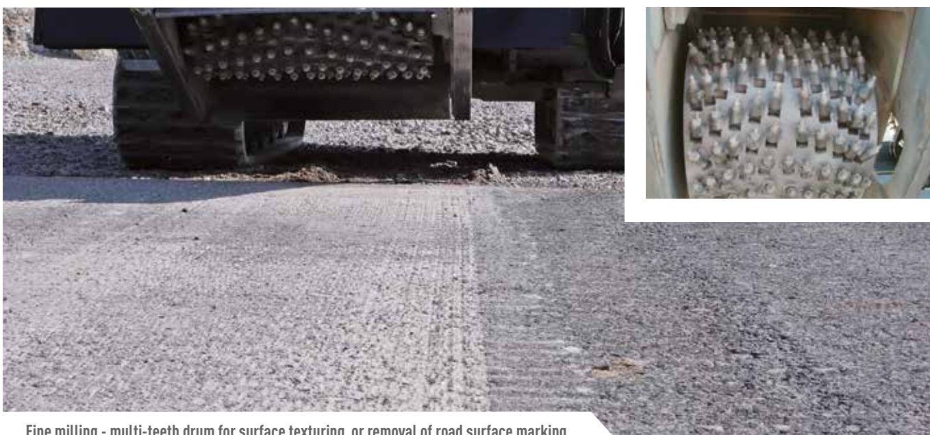
Fine milling - multi-teeth drum for surface texturing or removal of road surface marking.
